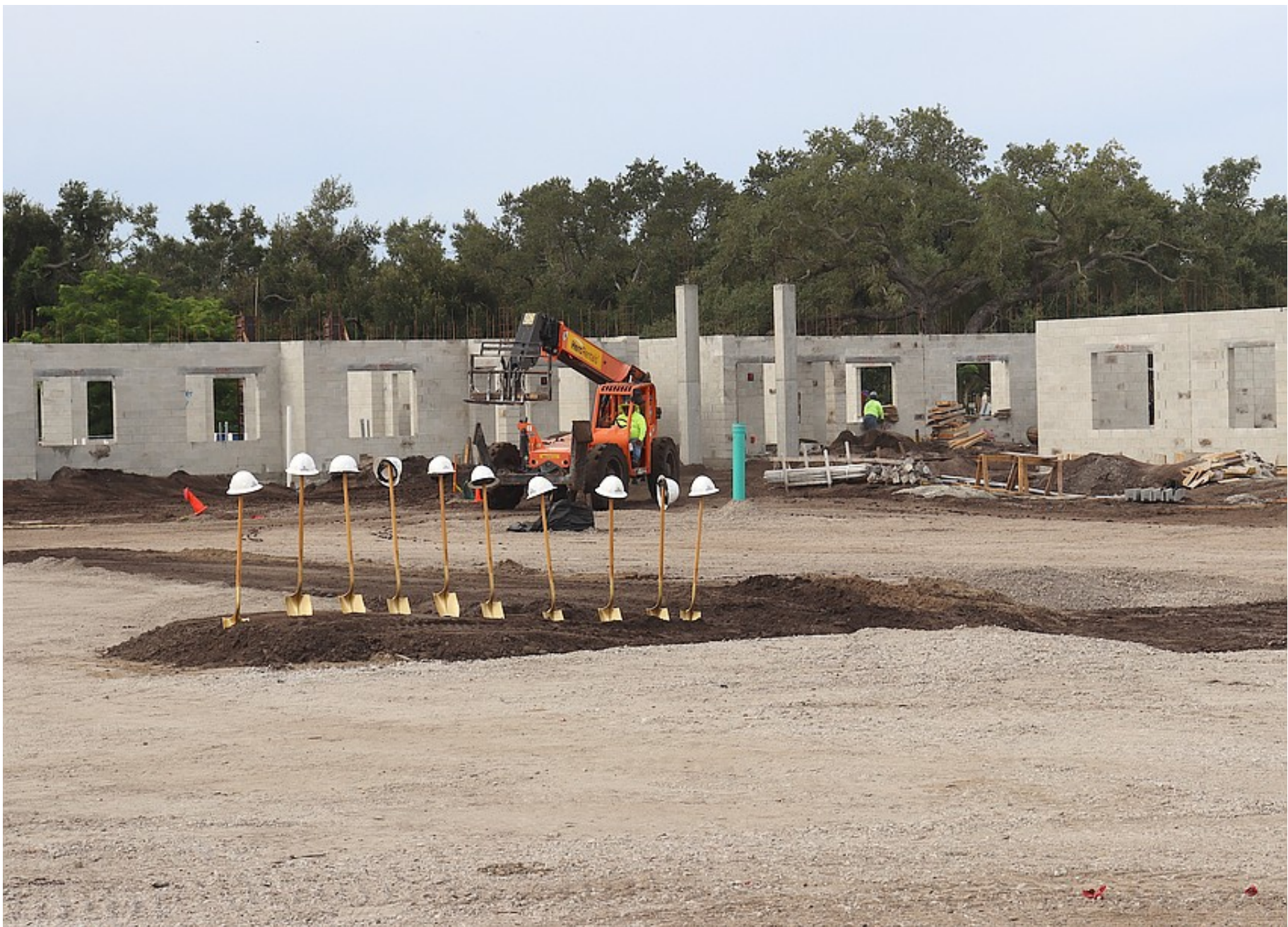
Construction is already well underway on Sarasota Housing Authority's Cypress Square II as it surrounds the ceremonial groundbreaking site. Photo by Andrew Warfield
