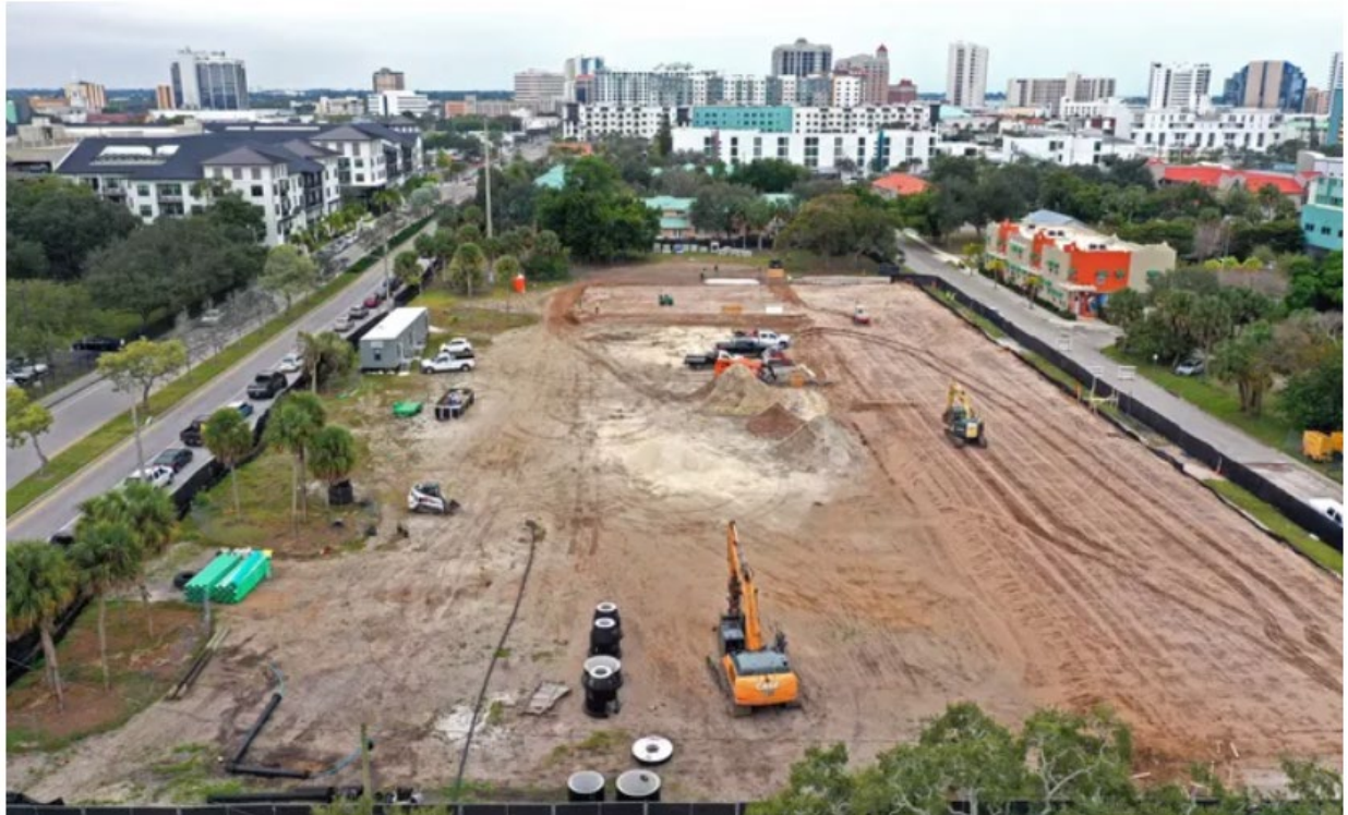
The construction site of Lofts on Lemon, an affordable housing development in downtown Sarasota. THOMAS BENDER/HERALD-TRIBUNE
